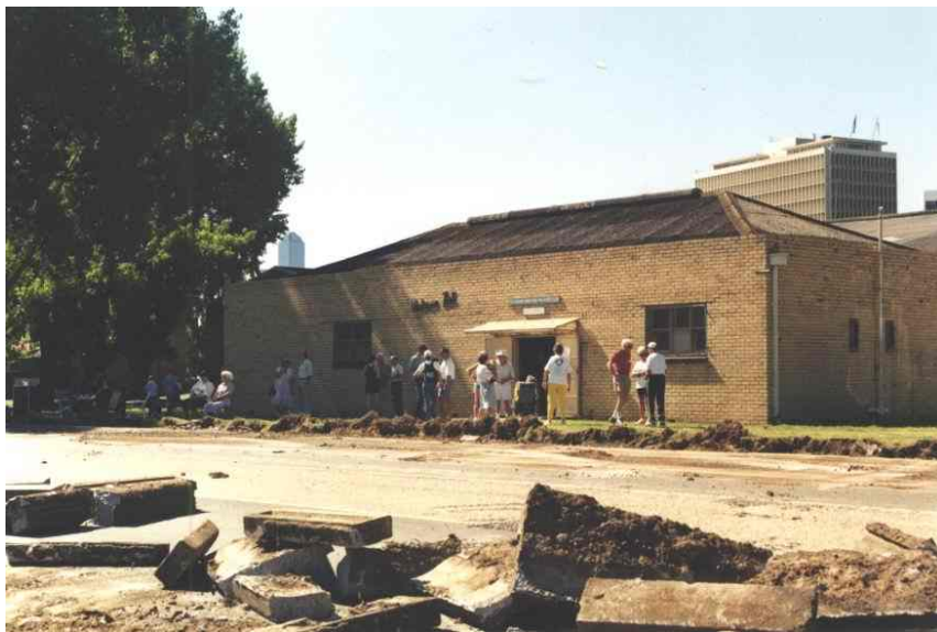
The final wake – with Lakeside Drive already being demolished – and the clubrooms soon to follow
